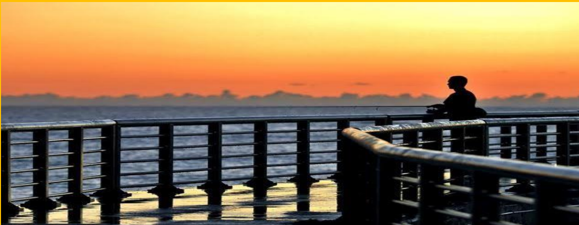
Sebastian Inlet Pier
